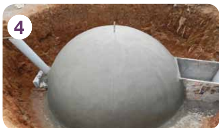
4 The manure inlet pipe (left), methane outlet pipe (top) and waste outlet shoot (right) are added
