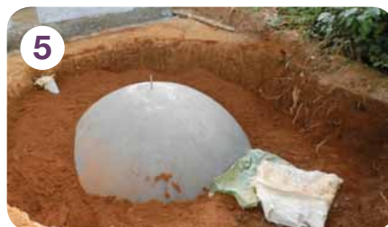
5 The structure is covered in earth
