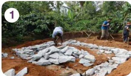
1 A hole is dug to house the biogas dome, and foundations are laid nearby for a simple cowshed
