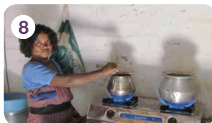
8 A pipe is attached to the top of the dome outlet, which leads into the household to supply the methane directly to a simple gas stove
