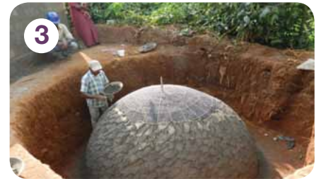
3 Three layers of concrete are applied to the dome to form a digestion chamber
