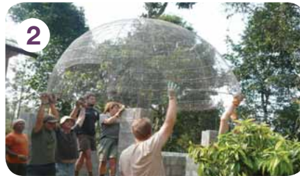
2 A large dome is handmade from wire and lifted into the hole
