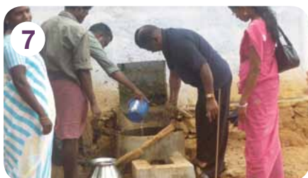
7 An inlet station is made, where the manure is mixed with water and then poured into the digester to start reacting
